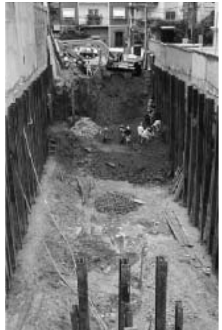
Digging the foundations
