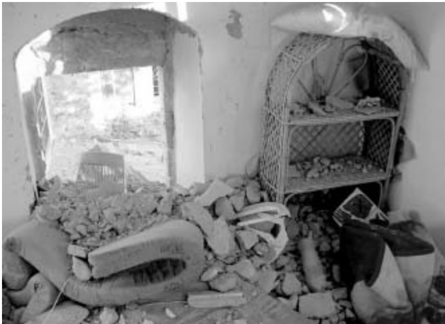
Destruction in Tzfas
