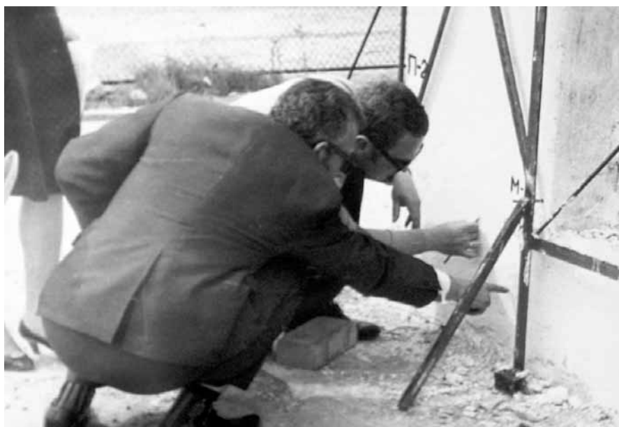
Aharon Grossman checking buildings after a controlled explosion to simulate an earthquake
